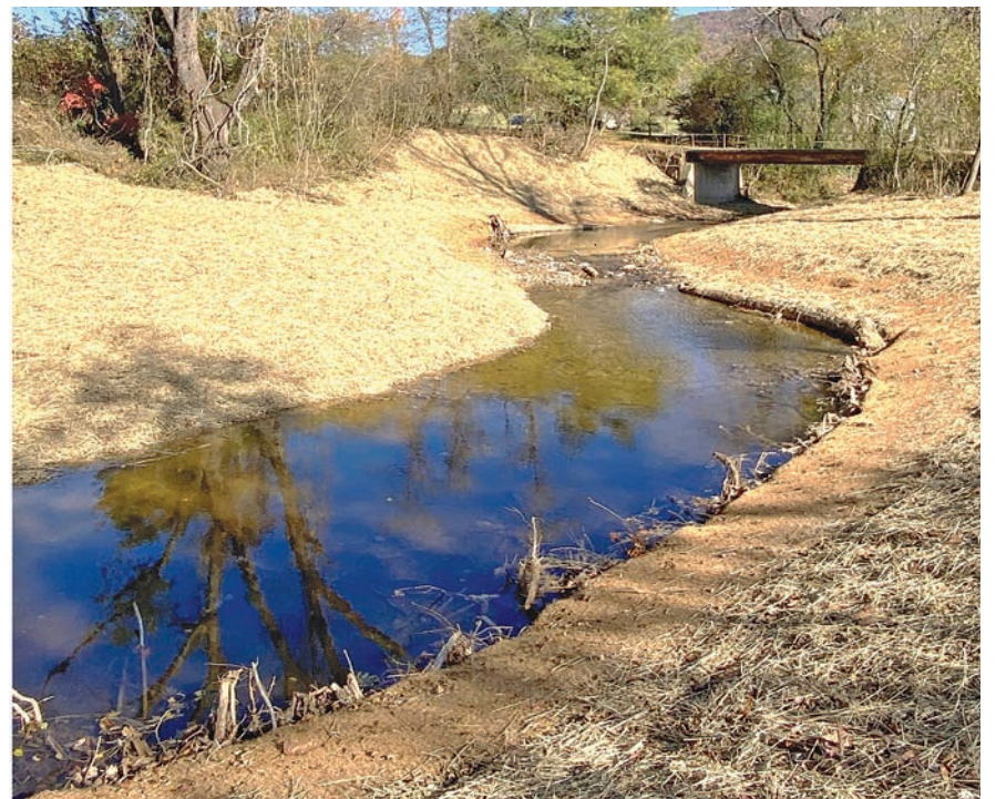
The brush toe technique protects the erosion-prone bottom of the near bank by anchoring stumps and roots all along the water’s edge. Layers of straw and coconut fiber fabric reduce erosion on the upper slopes while new vegetation gets started.
